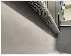
Figure 9 – Parapet internal TPO guttering with welded cap flashing and cladding cavity closure vermin strip.
