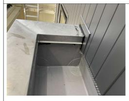
Figure 10 – Parapet internal TPO guttering with welded cap flashing and cladding cavity closure vermin strip. (Alternate view)
