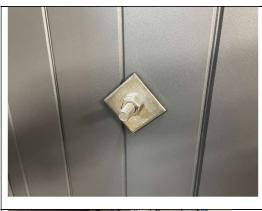
Figure 8 – Fixing penetration.
