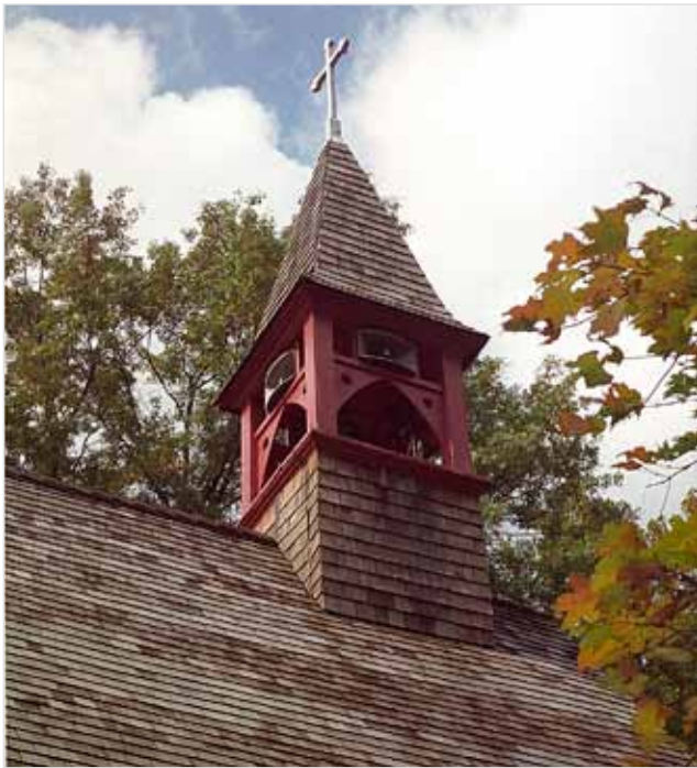
Figure 4. Thirteen-year-old shingle roof with random-width shingles.
