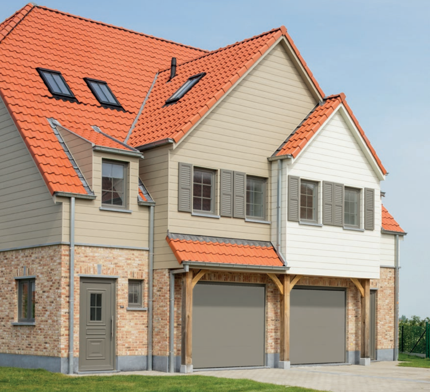
Top gable roof
