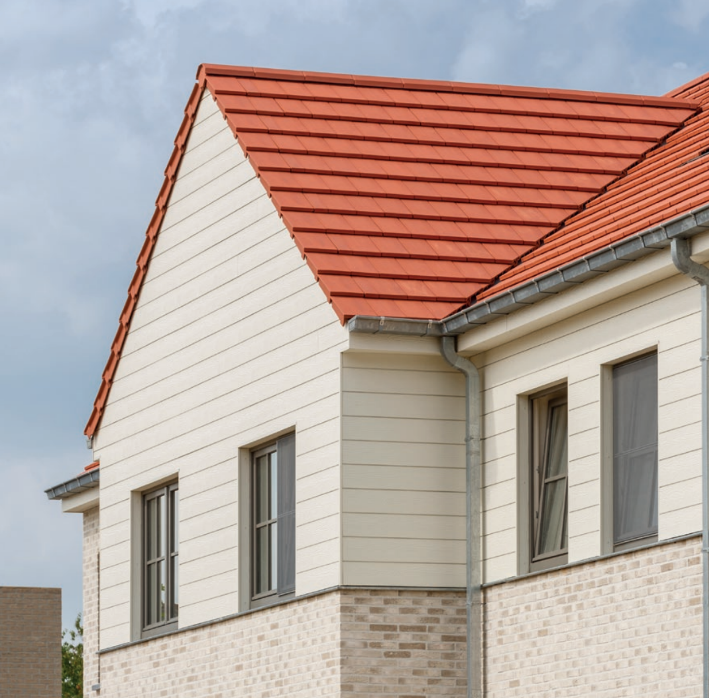
Top gable roof
