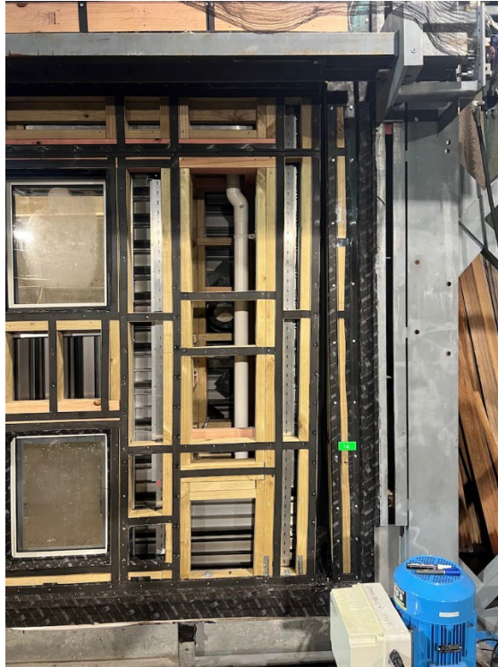
Figure 8: Photo of specimen racking at maximum extent, showing gap at bottom of jamb stud.
