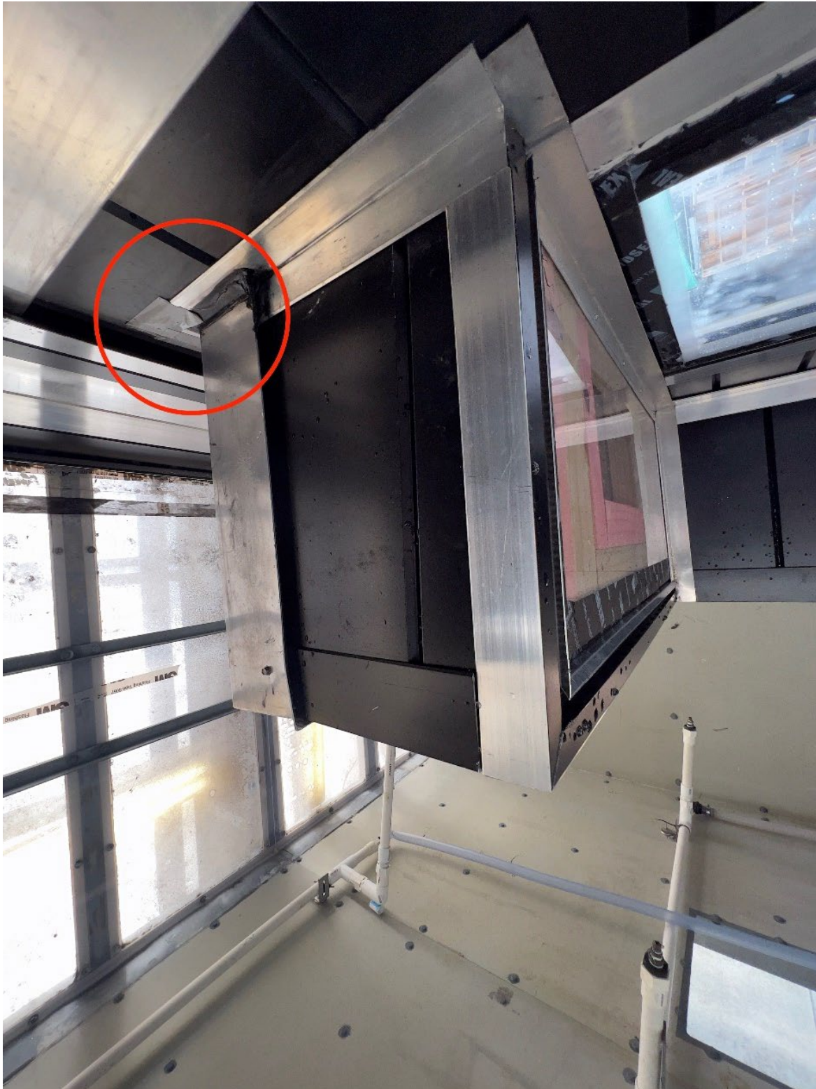
Figure 5: Parapet- sealed to remove from the test
