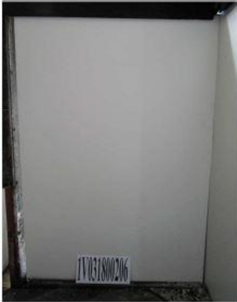
Before test (Long wing)
